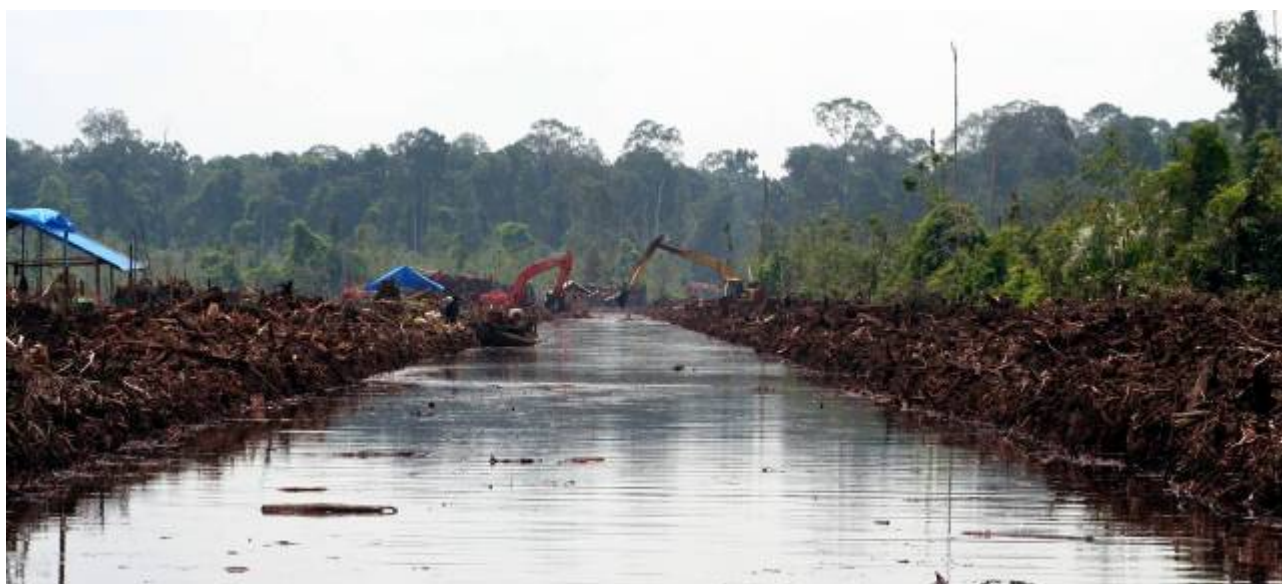
Canal opened for acacia plantation development and natural peatland forest waiting to be cleared in the background, Riau. © WWF Indonesia
