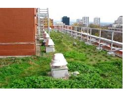
Above: Ecoroofs replace conventional roofing with a living, breathing vegetated roof system. This type of roof significantly decreases stormwater runoff, saves energy, reduces pollution and erosion, and helps preserve fish habitat.
