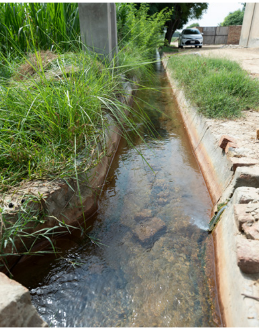
A 200 m watercourse lining project implemented by WWF at a farm in Multan, Punjab, Pakistan.
